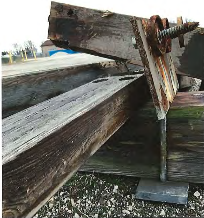
1) Side photo of Metal Connectors including Lag Bolts, Split Rings, and Plates
